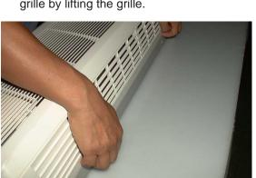
② Remove the fixing tabs (3) at the bottom of decorative grille.
